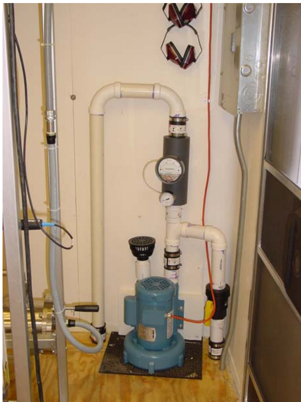
Figure II-3. Blower system for packed tower.
