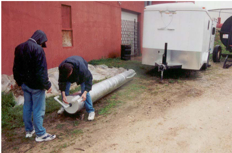
Figure II-2. Packed tower system being set up at site.
