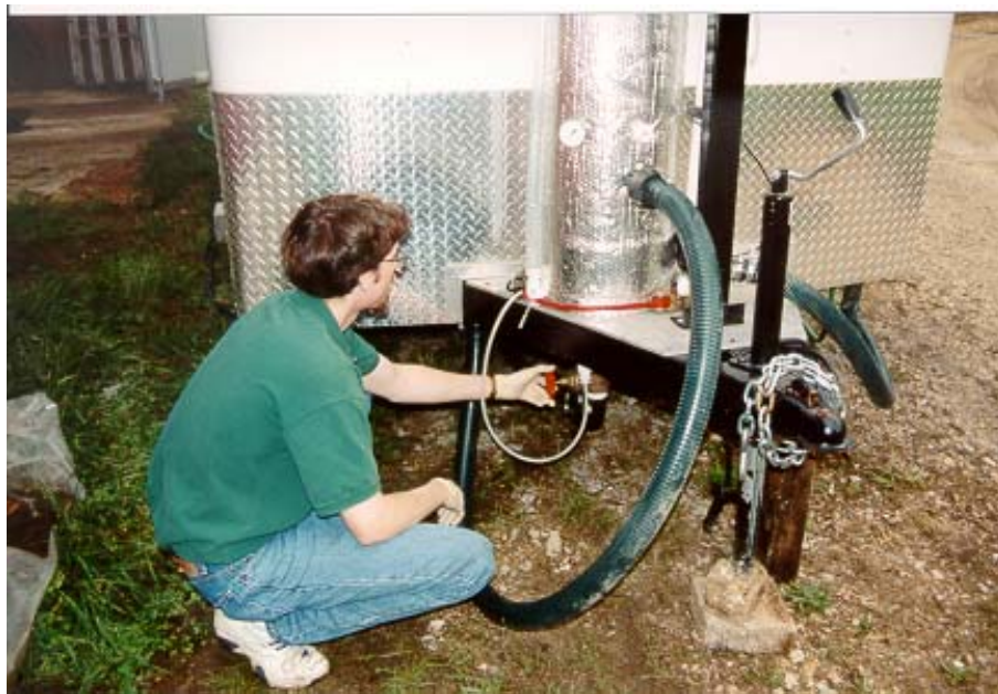
Figure II-4. Air and water connections at base of packed tower.
