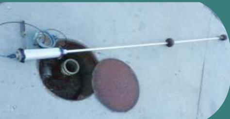
**If you have an automatic tank gauge, a qualified technician will have to remove the probes, inspect for residue, confirm the float(s) are moving freely and cables are free of kinks, etc.**
