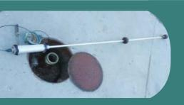
If you have an automatic tank gauge, a qualified technician will have to remove the probes, inspect for residue, confirm the float(s) are moving freely and cables are free of kinks, etc.
