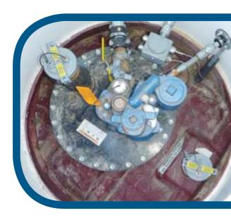
Containment sumps should be inspected and cleaned before starting any test. If a sump has a crack or its seals are loose, you may want to repair or replace it <u>before</u> spending money for a test.
